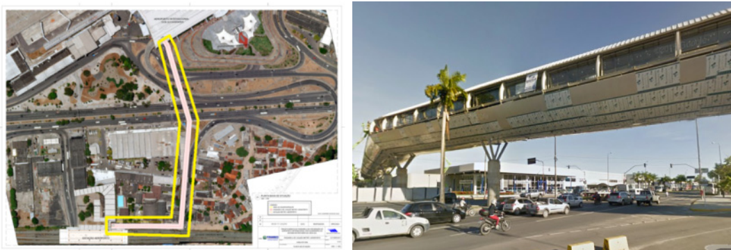
Figure 2. a) Aerial (left) and b) terrestrial (left) image of the walkway connecting the Guararapes International Airport and metro station. Source: Government of the State of Pernambuco
