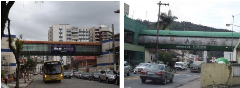
Figure 3. Rio Branco College (left) and Unimed Hospital (right), Blumenau-SC
